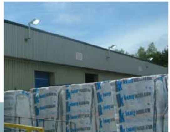
Outside Lighting - 1500 Watt Metal Halide
